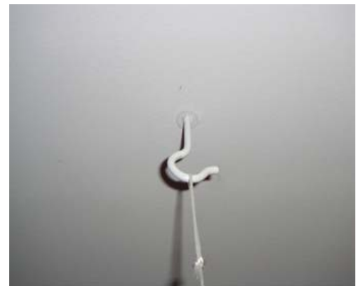
Screw Hook into Drywall Anchors - Attach loop of string
